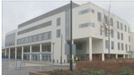
The new £225m, 512-bed hospital for west Kent with single rooms and en-suite facilities for all patients. Built under a private finance initiative, it will cost £20m a year for the next 30 years.
